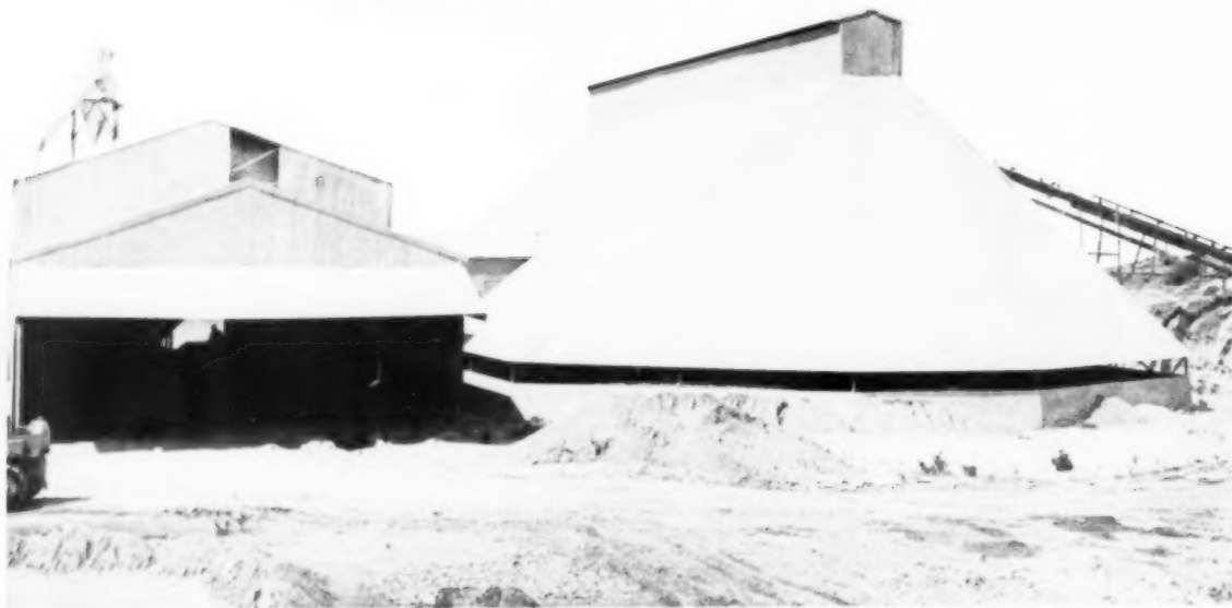
Varco Clay Storage Building at Payne Brick Company, Elgin, Texas
